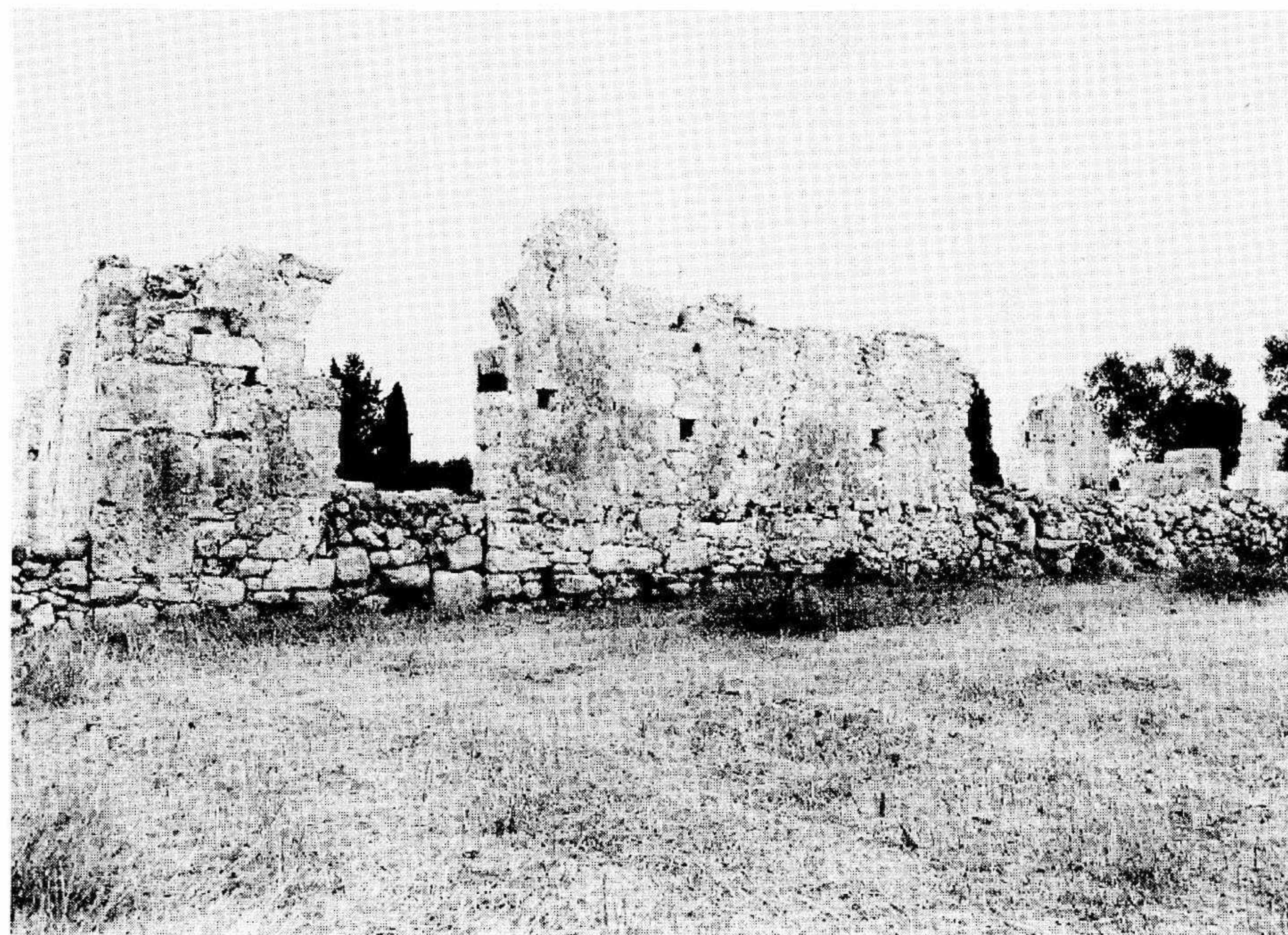
FIG. 10. Le Centoportre. View of the southern exterior wall. Note the blocking of the side entrance to the narthex. (Photo by Paul Arthur)
